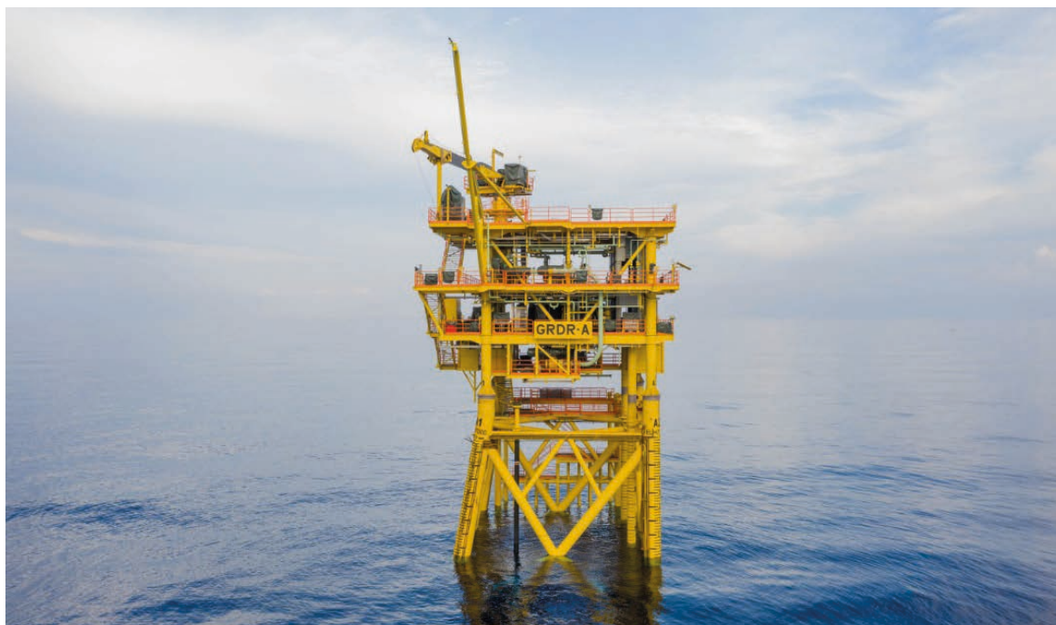
FIGURE 1 SMEP's first fully renewable-energy powered offshore platform, Gorek, achieved its first gas in May 2020.
