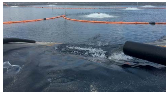
Shell's Salt Water Disposal (SWD) facility in Permian Asset in West Texas, (USA).
