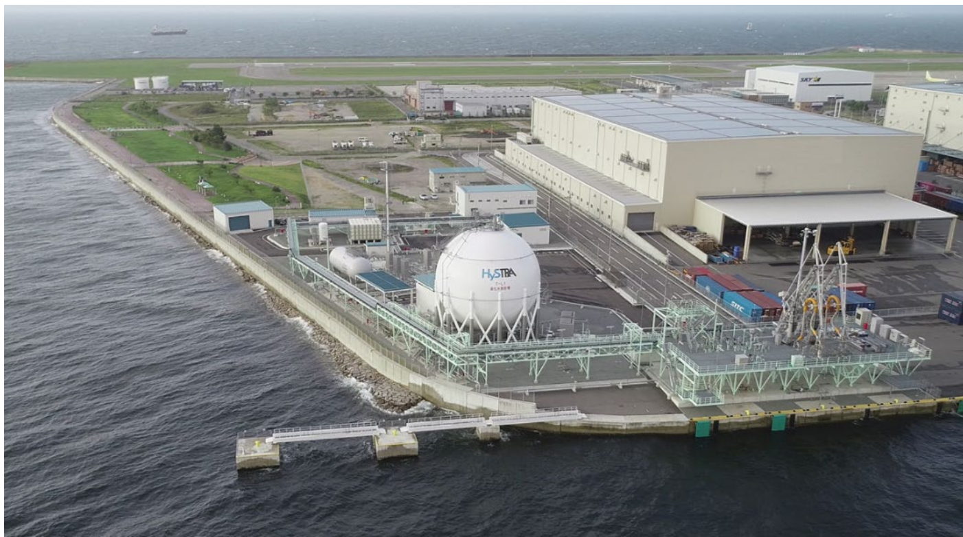
FIGURE 4 The vacuum-insulated LH 2 storage tank in Kobe.
