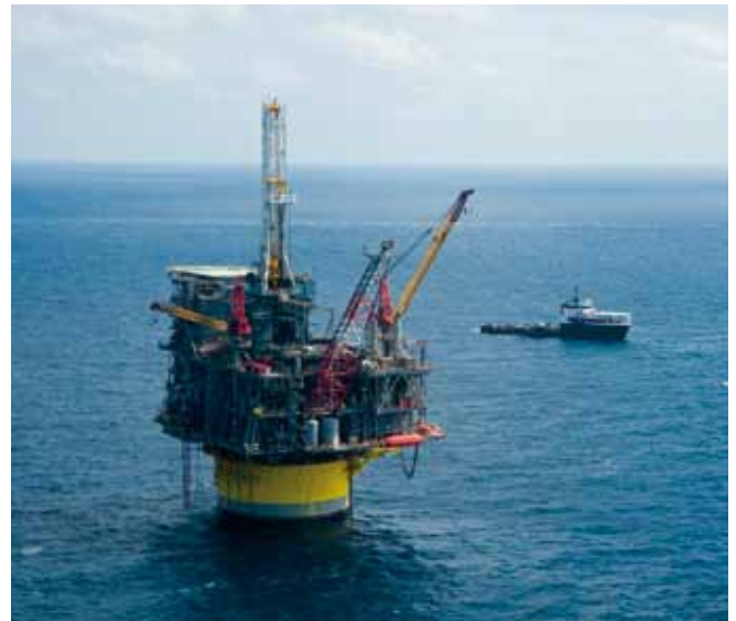
Perdido deep water project, Gulf of Mexico, USA, 2010
